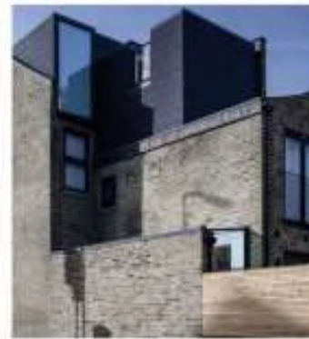
Retrofit of an Edwardian house London, United Kingdom
